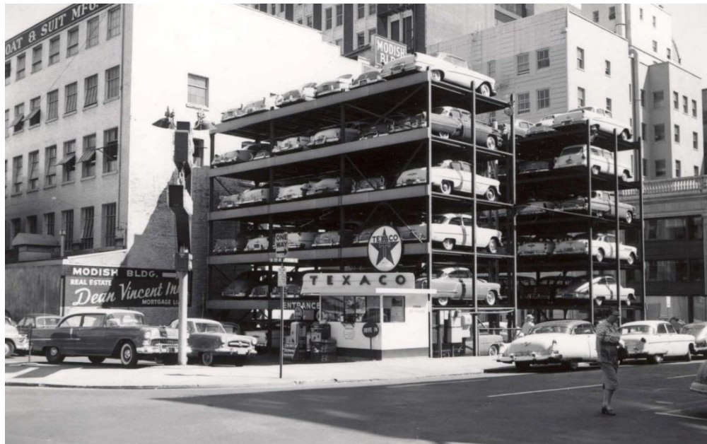
Fig.4. The very first mechanized parking in the world
